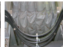
There are also jumper wires connecting rolling stock
