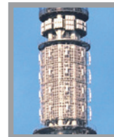
Antennas on the Tokyo Sky Tree
