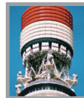
Face-sharing omni-directional multi-panel antenna array on Tokyo Tower
