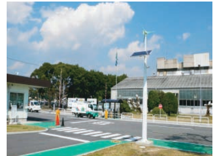
Wind and solar powered lighting
