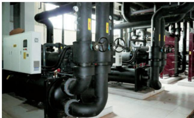
Switched from coal boilers to heat pump equipment for heating and preventing atmospheric pollution
