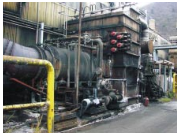
Smoke-extraction desulphurization equipment
