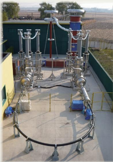
High-temperature super-conducting power cables
