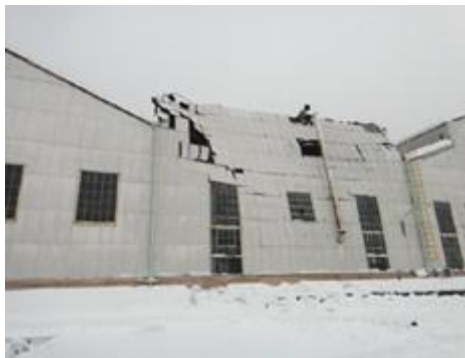
Collapsed roofing immediately after the snow damage
