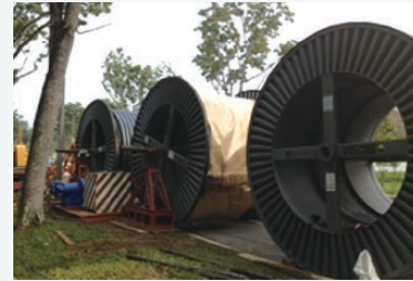
Laying site of ultra-high voltage power cables
