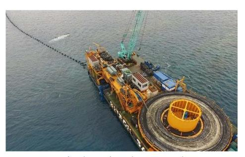
Laying submarine water pipes
