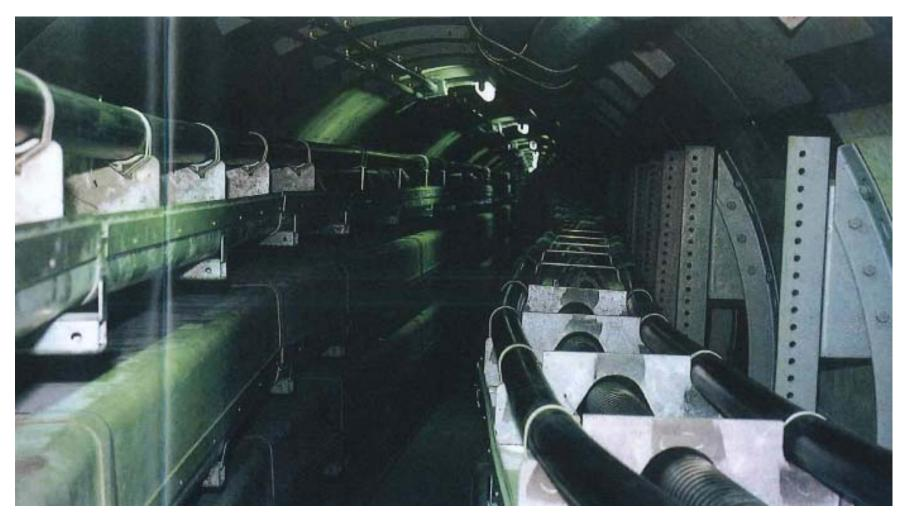
Ultra high voltage cable installation example (Inside the cable tunnel)
