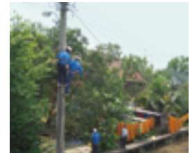
Installation of optical fiber cable overseas
