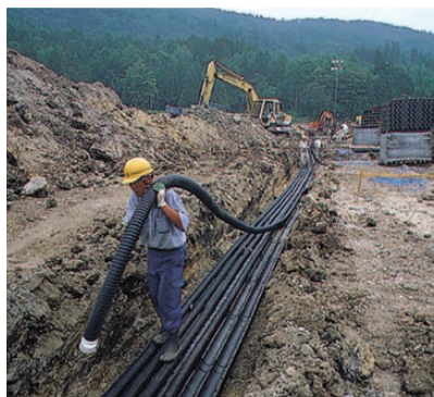
Long, continuous laying
