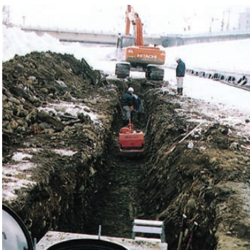
Backfilling with produced soil
