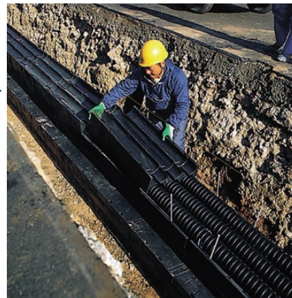
Laying work without using heavy machinery
