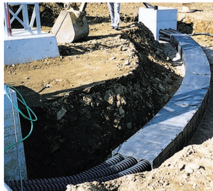
■ Making a horizontal detour around an obstacle
