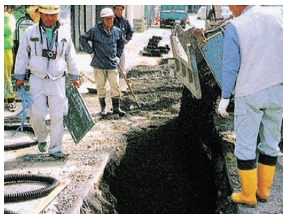
■ Underground installation crossing a road
