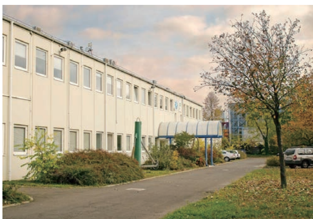
Figure 1 The building of FETI in Budapest, Hungary where all the offices and laboratories are located.
