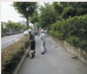
▲ Cleaning activities around the works
