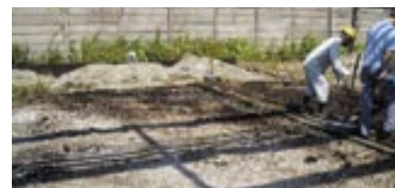
Chiba Works / Work of replacing soil
