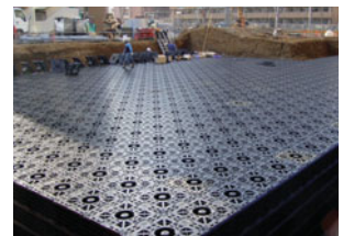
Rainwater retention and infiltration system based on resin block assembly method (HYDROSTAFF)
