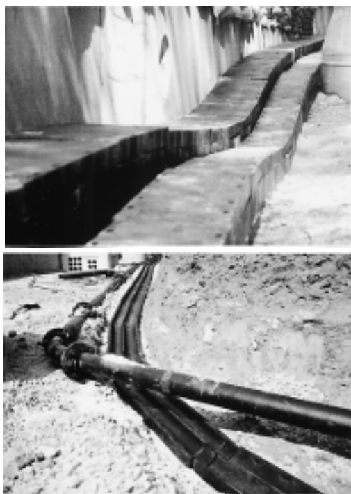
図7 曲がり管路の敷設 Laying of curved lines
