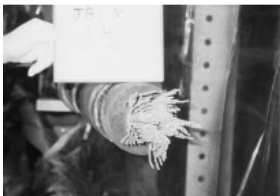
写真4 素線絶縁導体の皮膜除去 Film removal of insulated strand conductor
