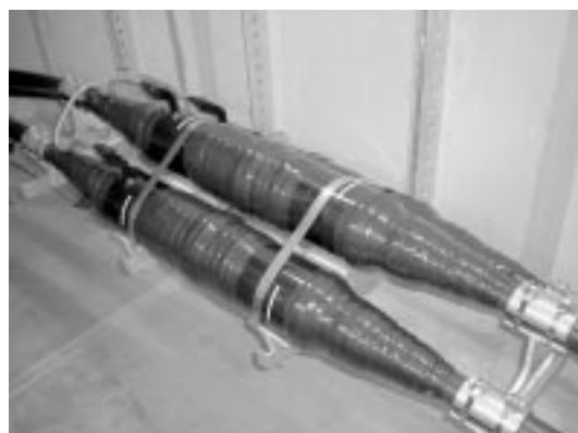
図8 66 kV CSJ組立状況 View of 66-kV CSJ on site
