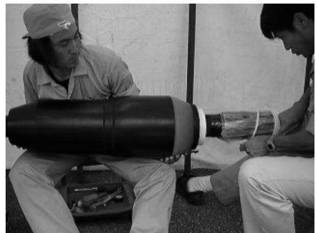
写真4 CSJ組立て作業風景 Assembling CSJ on cable (Only pulling spiral-core completes assembly)
