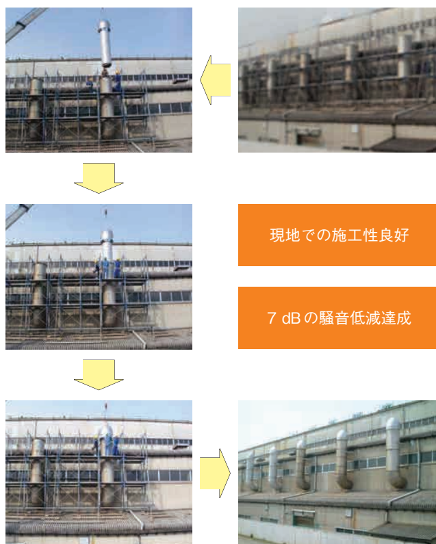
図19-2 排気筒の施工風景 Installation work of sound absorber.
