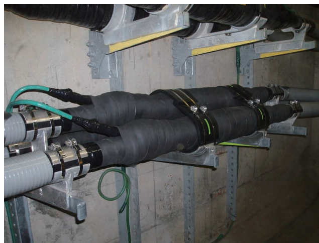
図3 ERJの現地据付状況 View of assembled ERJ on site.
