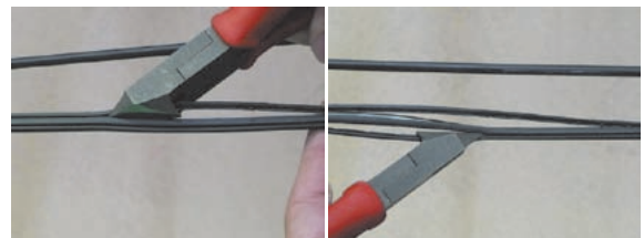
図2 連結部を斜ニッパにて切断 Cut the connection part with a nipper.
