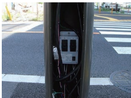
図2 電源ユニット取付け状態 Installed water-proof type circuit breaker with switchboard function.
