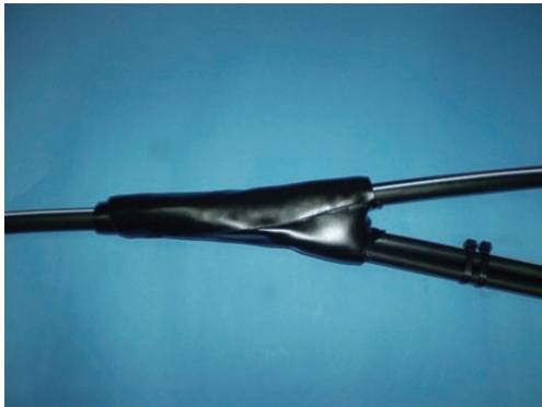
図7 粘着カバー処理 Adhesive protection covering process.
