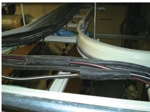
図3 敷設状況 Installation situation.
