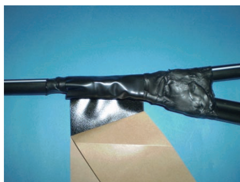
図6 絶縁シート処理 Insulation seating process.
