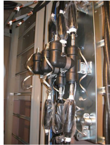
図5 h分岐本体との接続 View of connecting process.
