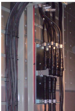
図1 h分岐縦幹線仕様敷設状況 View of assembled joint.
