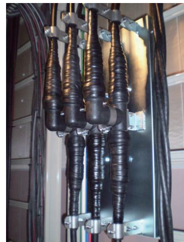
図6 完成品 View of assembled joint.
