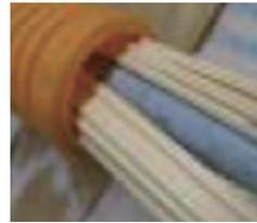
30 cables in the pipe of 22 mm in inner diameter at once
