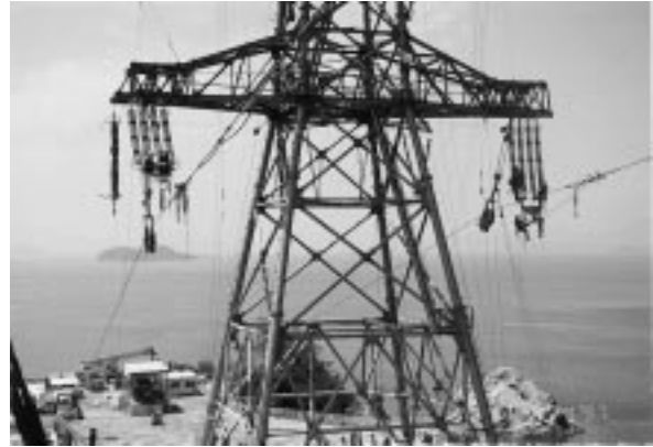
Photo 2 Tensioning at tower No. 8
