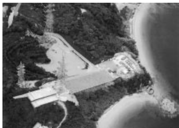
Photo 1 No. 8 tower, drum yard and large inclined stages
