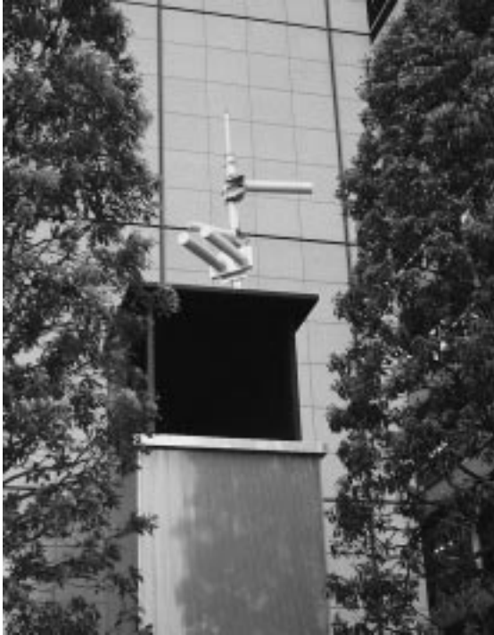
Photo 2 Outdoor antennas for base station (from top in order: sleeve antenna for 280-MHz pager, Yagi antenna with radome for 800 MHz, Yagi antenna with radome for 1.5 GHz, 2-tier stacked Yagi antenna with radome for 800 MHz band)
