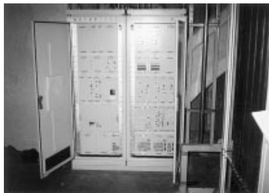
Photo 1 Appearance of central repeater station
