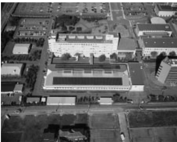
Figure 4 Solar photovoltaic system
