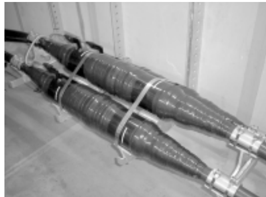
Figure 7 Assembled CSJ for 66-kV XLPE cable
