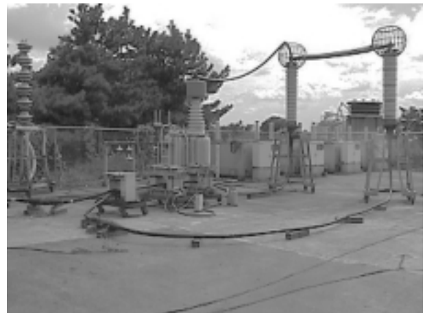
Figure 10 Long-term test of 66-kV CSJ
