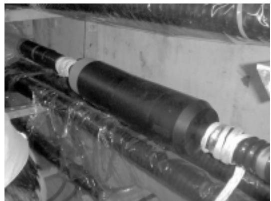
Figure 5 Assembled CSJ for 110-kV XLPE cable
