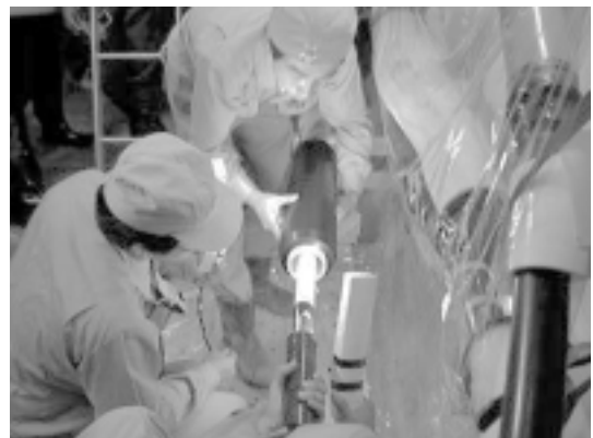
Figure 6 66-kV rubber unit inserted onto cable
