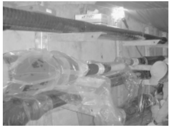
Figure 4 110-kV rubber unit inserted onto cable
