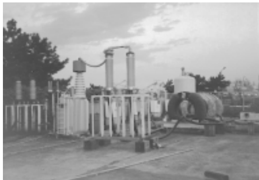
Photo 1 Long-term aging testing of 66-kV termination with composite hollow insulator
