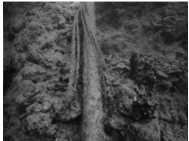
Photo 1 Submarine cable laid 28 years ago.
