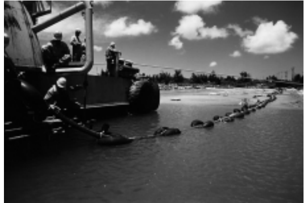
Photo 2 Cable landing on Miyakojima.
