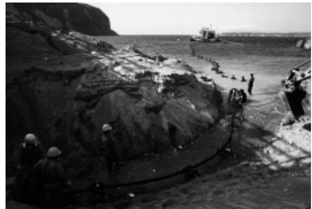
Photo 3 Cable landing on Niijima.
