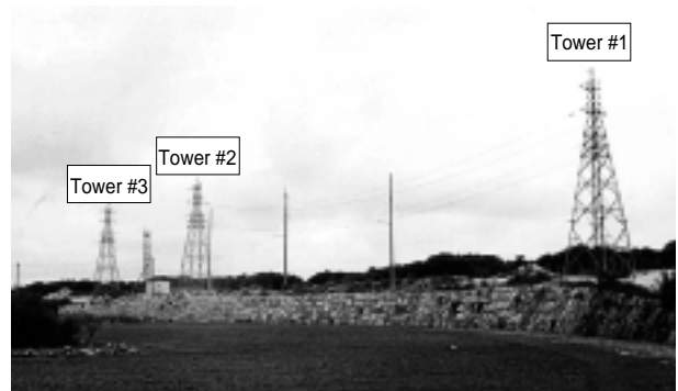
Figure 7 Miyakojima test line.
