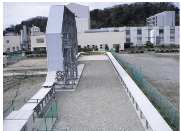
Figure 9 Test line of the 500-m HTS cable photographed from the termination.
