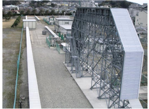
Figure 8 Test line of the 500-m HTS cable photographed from the U bend section (1).
