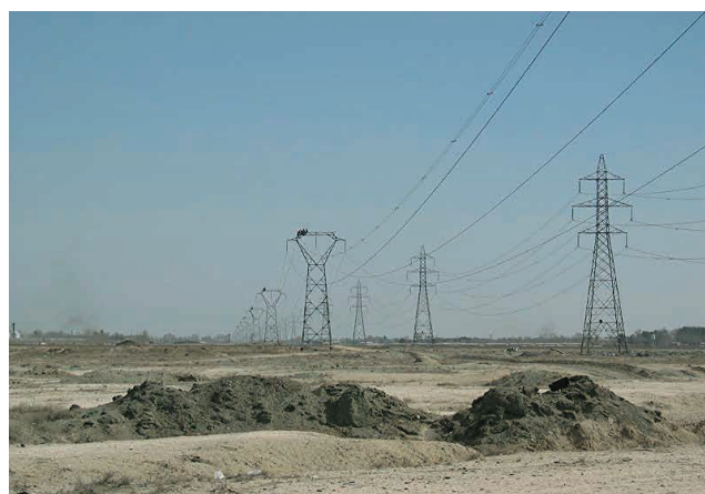
Figure 30 OPGW live-line installation for 220-kV power transmission line in Teheran, Iran.
