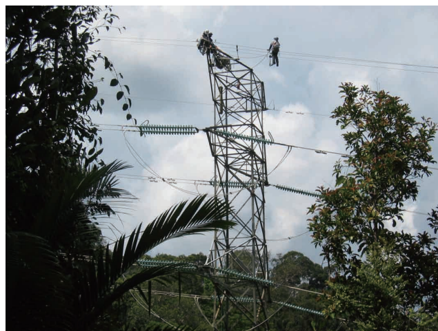
Figure 31 OPGW live-line installation for 275-kV power transmission line in TNB, Malaysia.
