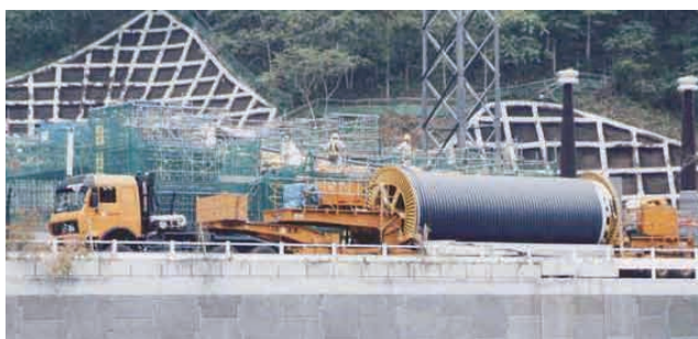
Figure 2 Installation of a long-length cable using a special-purpose vehicle.
