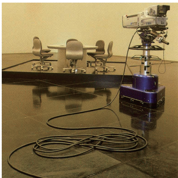
Figure 43 Optical fiber-composite TV camera cable system.
