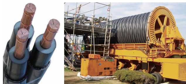
Figure 4 Large-sized Triplex-type XLPE cable and its installation.
