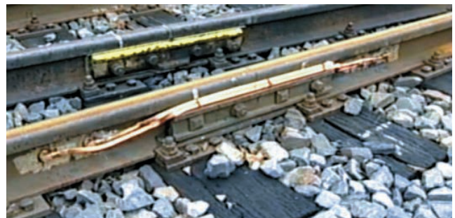
Figure 1 Rail bond installed on a rail.
