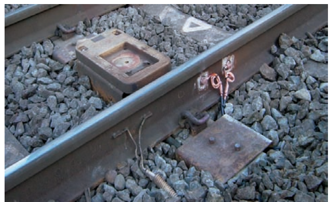
Figure 2 Signal bond installed on a rail.
