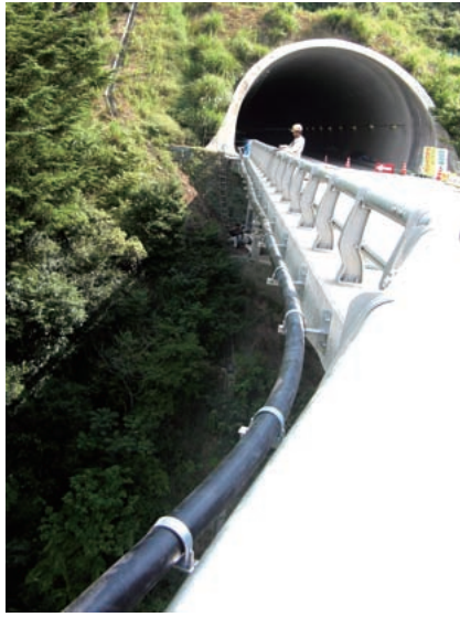
Figure 5 Installation in tunnel as fire-fighting piping.
