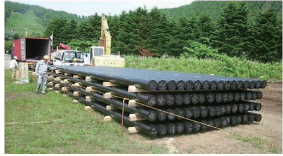
Figure 4 Supply in straight pipe configuration (AQX-VR).
