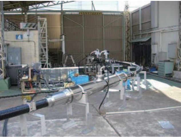
Figure 8 Short-circuit current test of the 66 kV-3 kA YBCO HTS cable (A cable joint, and a 10 m cable that was set in the back from the joint were fabricated by FEC).
