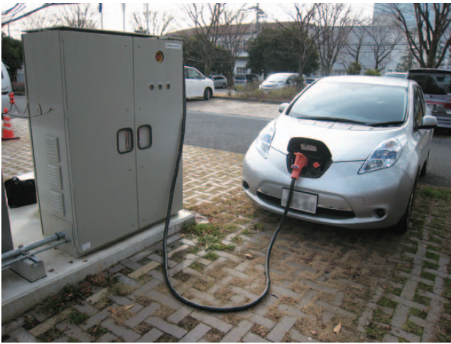
Figure 4 Electric Vehicle and a power conditioning system.
