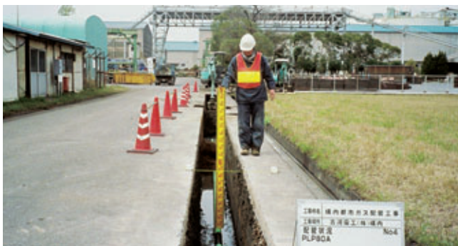
Laying a 2,000-meter city gas pipeline for switching fuel
