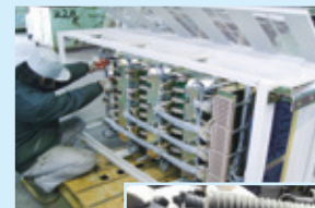
Discarded distribution boards
