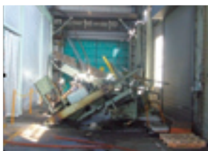
Fallen crane at the Nikko Works
