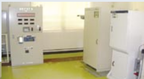
Automatic monitoring equipment for wastewater
