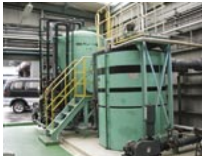
Facility for emergency treatment of rainwater
