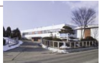
Front entrance of the Ueda Factory
