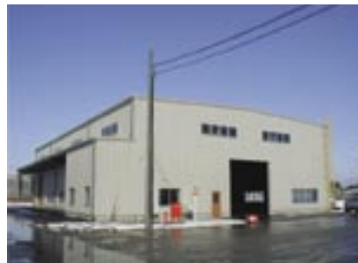
Wood work center
