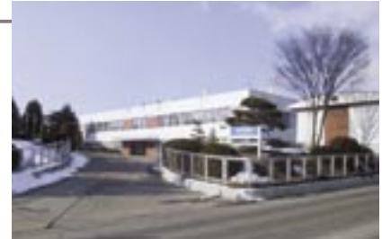
Front entrance of the Ueda Factory
