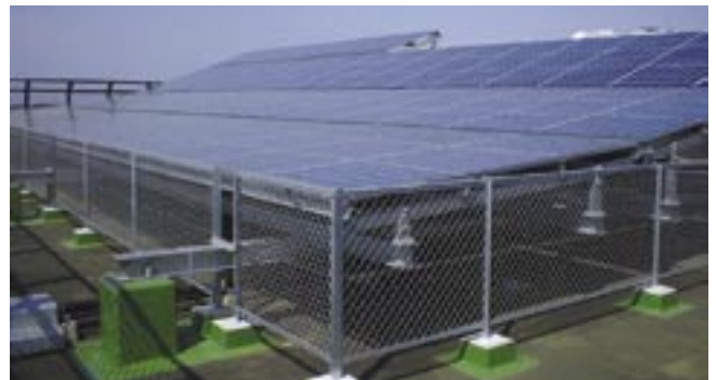
A 30 kW solar power system, installed by us on the roof of the Zushi Municipal Office (installation completed in February 2003)
