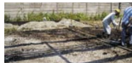
Chiba Works / Work of replacing soil
