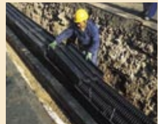
Cable duct for underground laying (KOHTA KUN)
