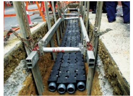
Example of the construction of a recycled duct guard
