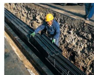
Cable duct for underground laying (KOTA-KUN)
