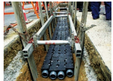
Example of the construction of a recycled duct guard
