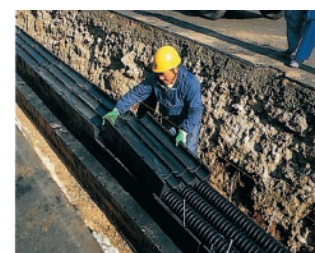
Cable duct for underground laying (KOTA-KUN)
