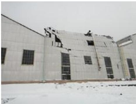
Collapsed roofing immediately after the snow damage
