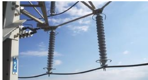
I-string assembly for jumpers
