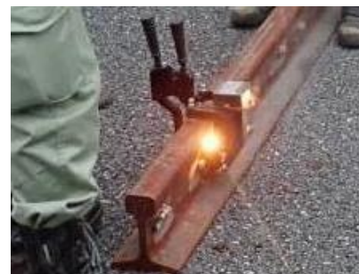
Welding using copper thermite
