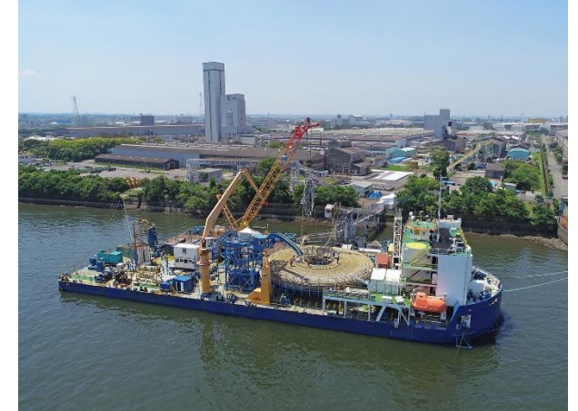
Loading submarine cable on a barge
