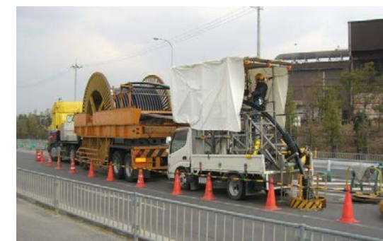
Cable installation worksite
