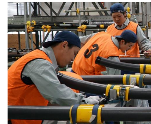
Installation skills training
