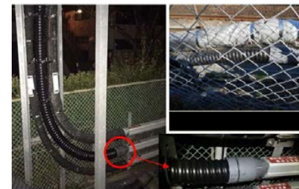
Conduit installation at a location where the cable rises vertically
