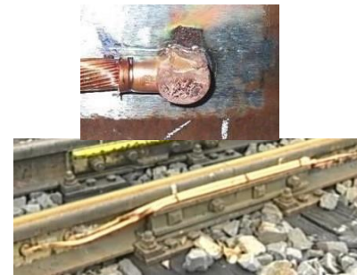
Rail bond made using copper thermite
