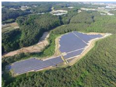
Kamata No. 1 Solar Power Plant in Hokota City
