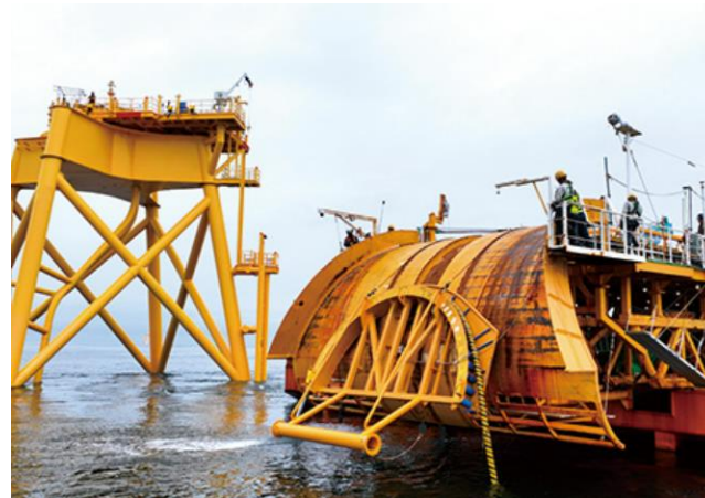
Installation worksite at the Ishikariwan Shinko offshore wind farm
