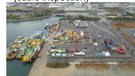
Image of spare submarine cable and stand-by repair barge service
