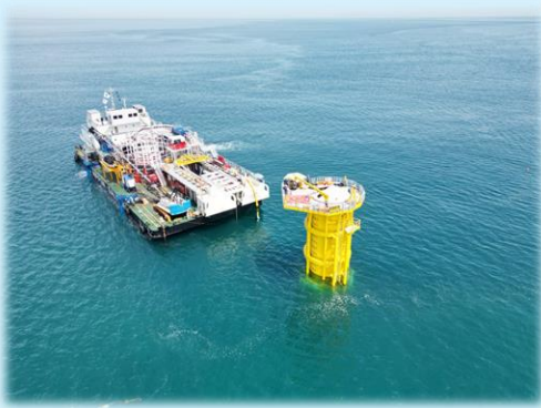
Ishikariwan Shinko offshore wind farm project- View of the cable laying operation (Photographs provided by Green Power Investment Corporation)
